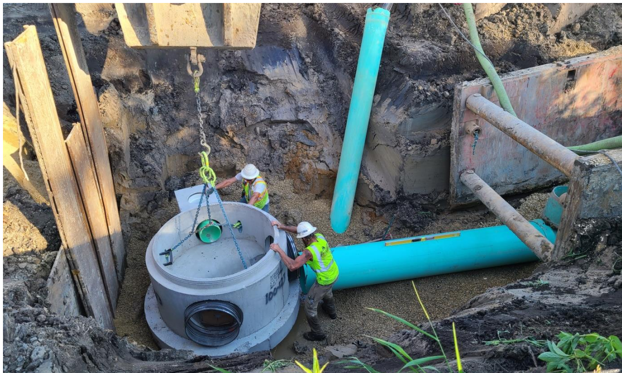
Figure 1: Crews Setting the Last Interceptor Manhole
