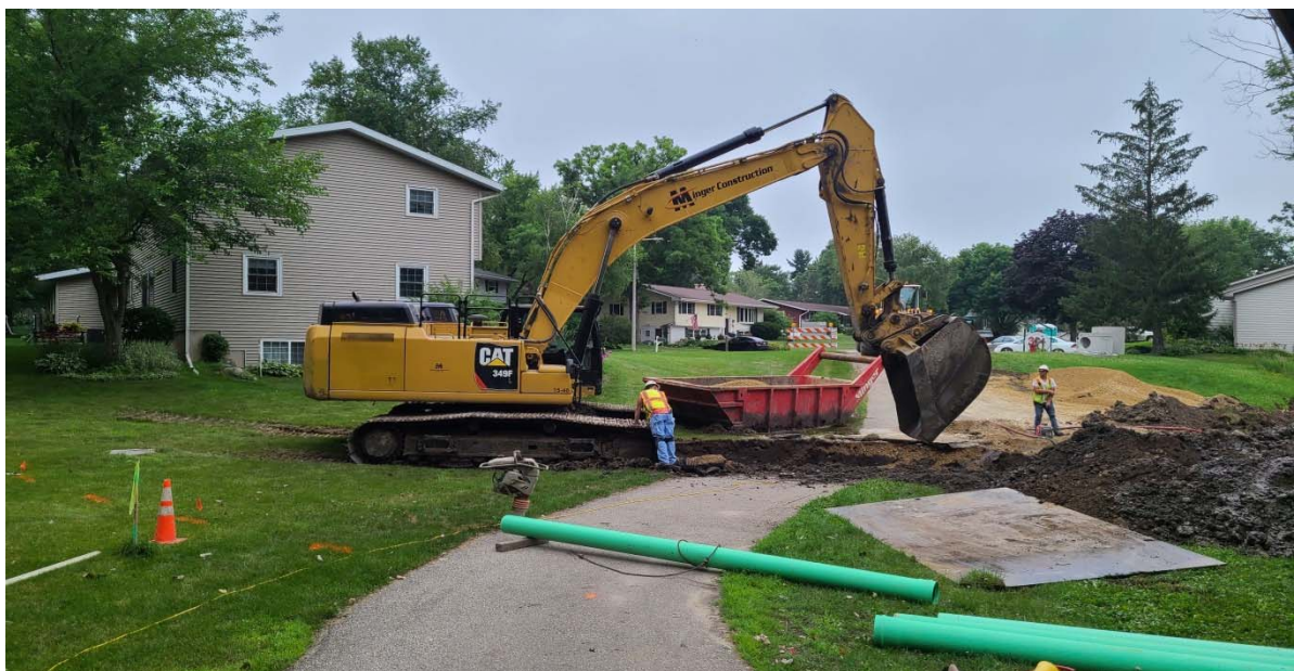
Figure 1: Crews Working on Lincoln Street Local Connection
