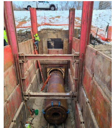
Figure 1: Interceptor Sewer Tunneling Launch Pit w/ 72-Inch Casing
