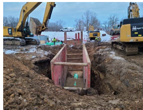
Figure 1: Pipe Installation South of S. Main St.
