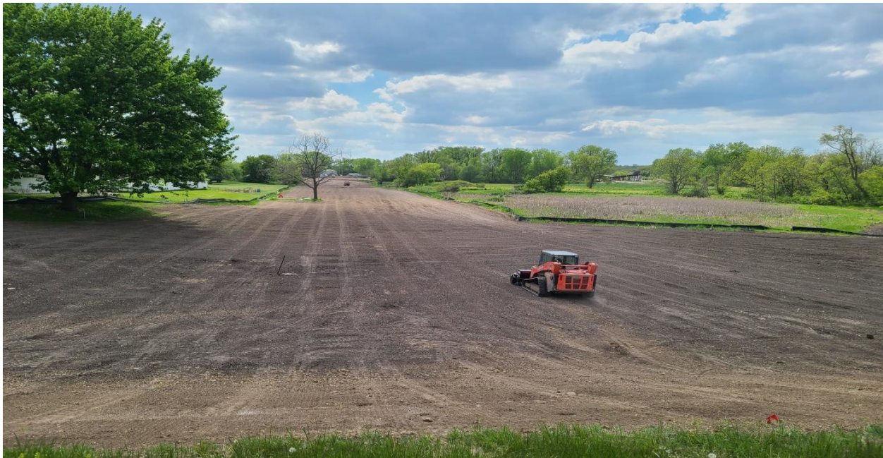
Figure 1: Grading and Seed Restoration from Bruce Street to Main St
