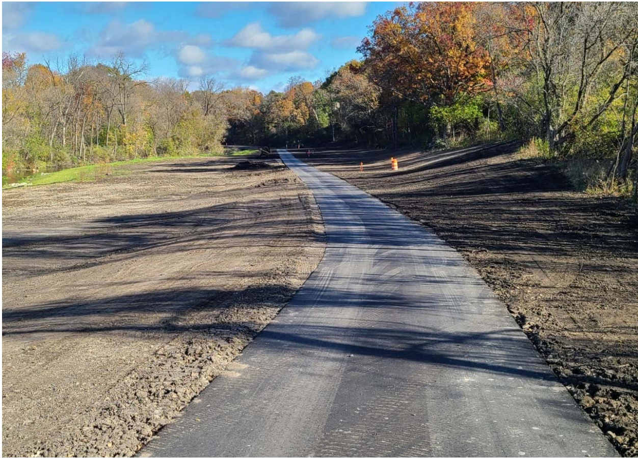
Figure 1: Final Path Grading
